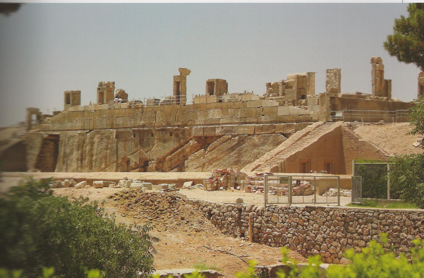
...quarters connected by staircase to Xerxes' palace on the terrace (at Persepolis)
